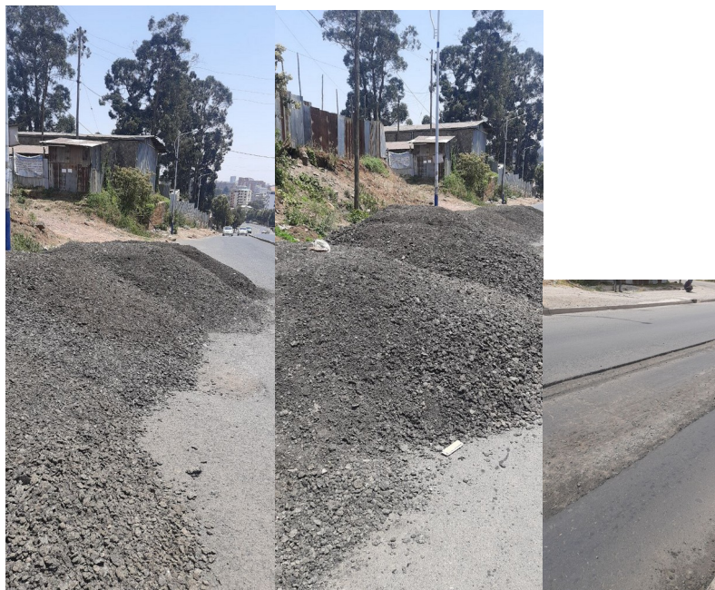
Figure 1 Source of RAP material from AACRA road project (photo taken during sampling)
